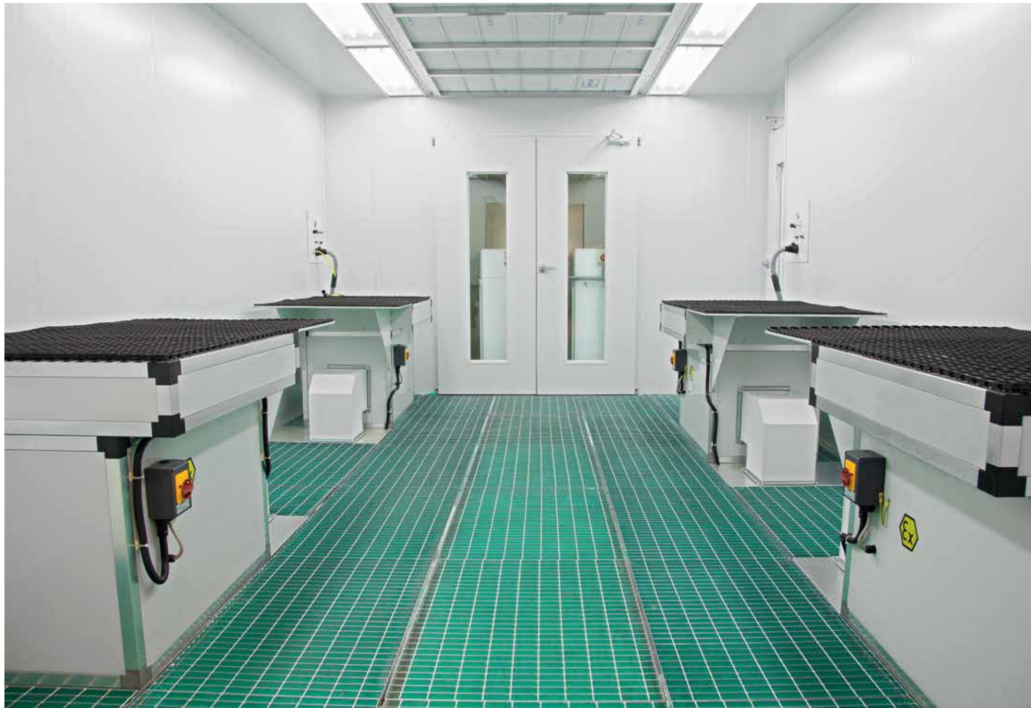
Carbon Fibre Processing - Italy
